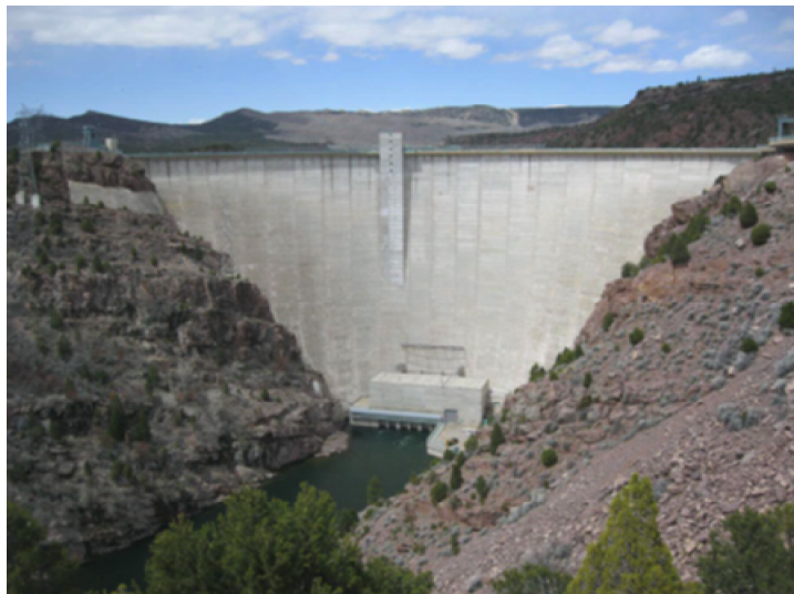
Figure 2-1: USBR's Flaming Gorge Dam and Powerplant
